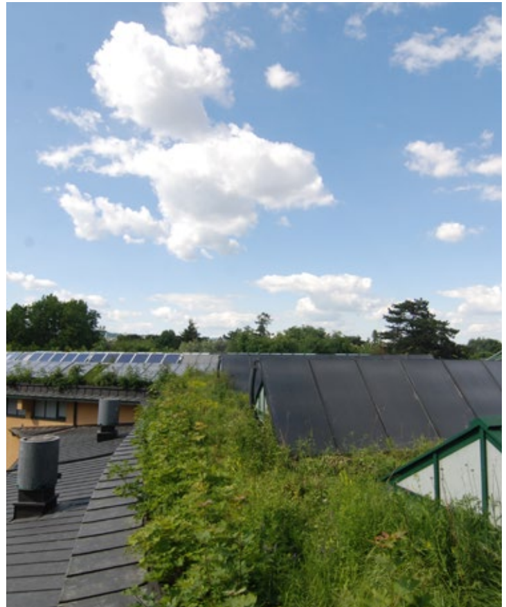
BOTTOM RIGHT: VIENNA ZOO, AUSTRIA A solar power plant installed on the roof of the elephant's living quarters produces around 90 megawatt hours of energy annually.
